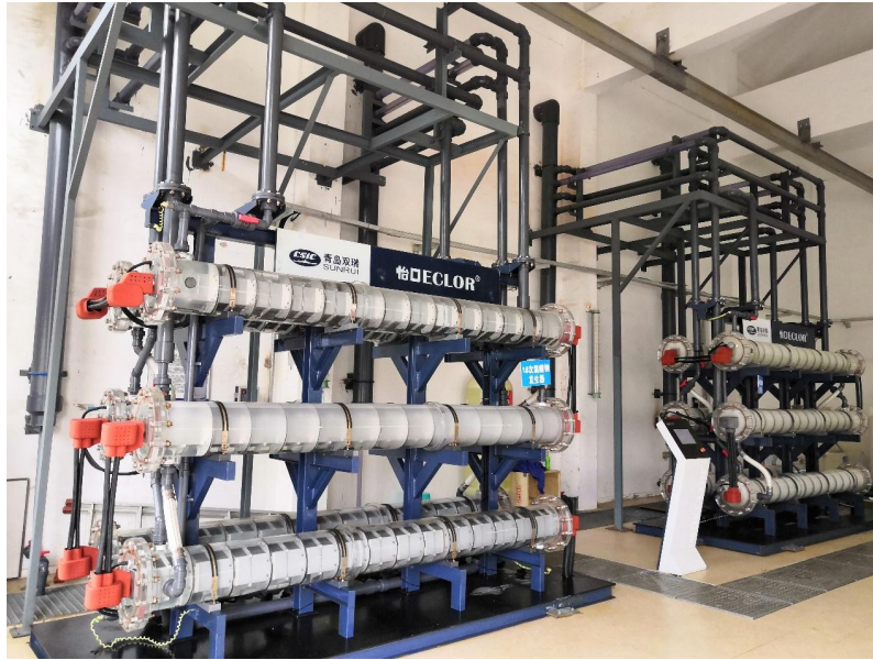
Jinhua Water Plant (Second phase)
