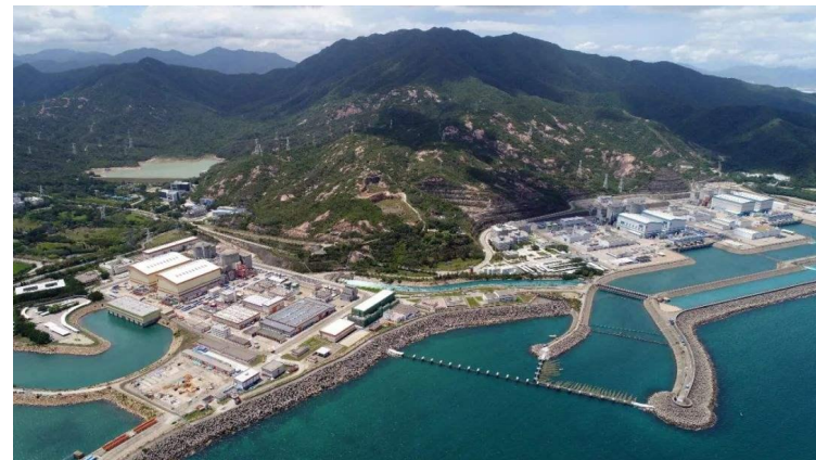
Zhangzhou Nuclear Power Plant
